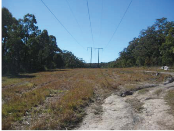
Photo 13: View to north along a powerline corridor
